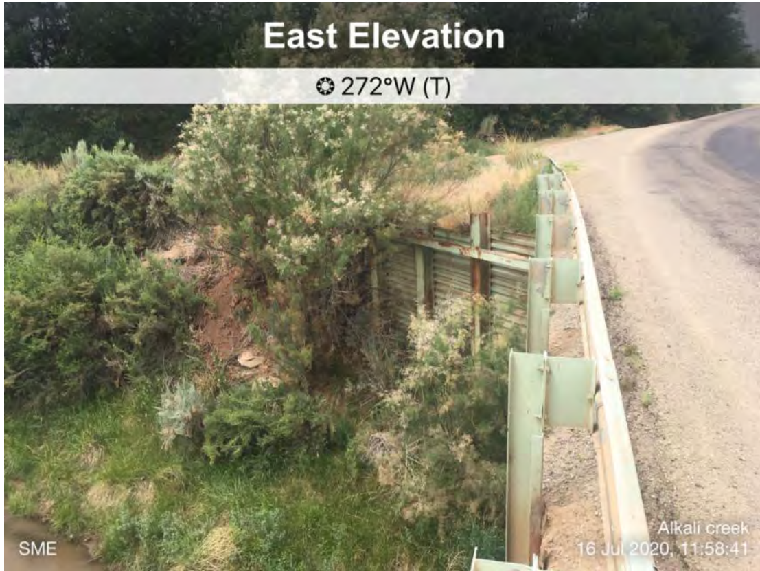
Description: Paint on guardrail and metal bridge structures (lead paint?)
