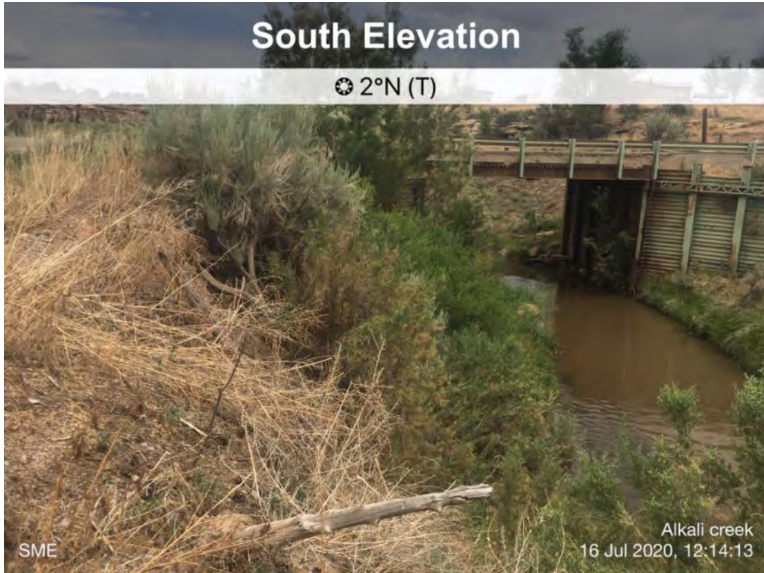
Description: General site characteristics
