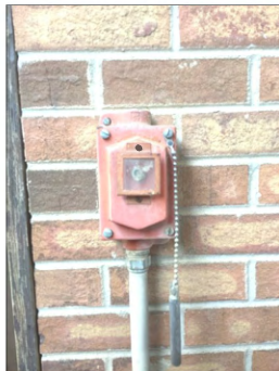
Outdoor alarm box is not operating.
